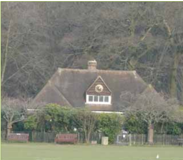
The cafe is popular with visitors but the kitchen facilities are restricted.
